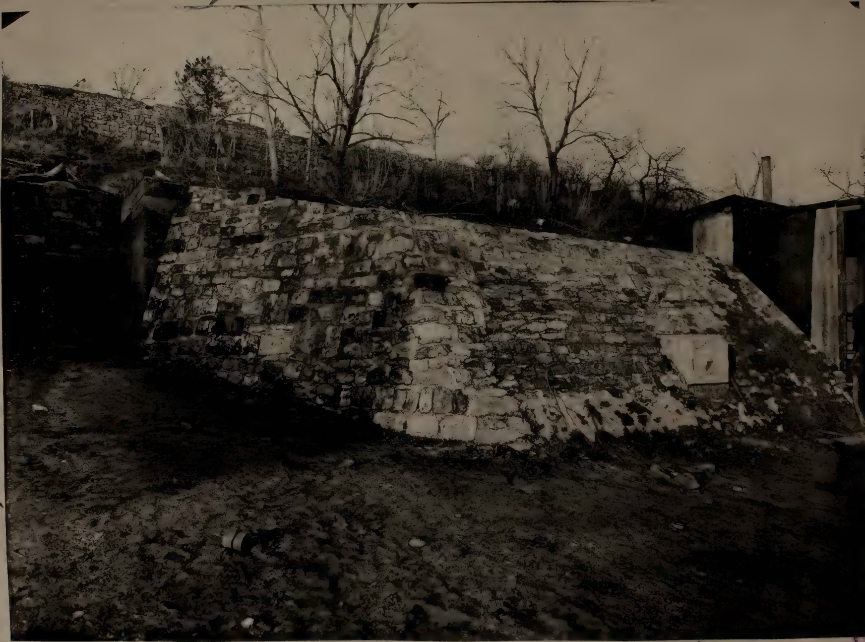
A typical German concrete and stone dugout.
